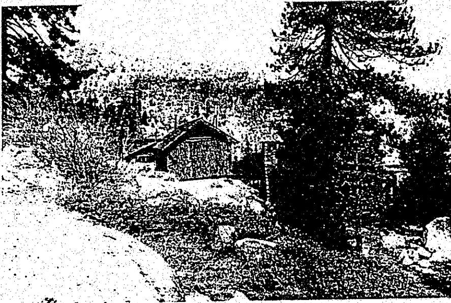
Cabin No. 71, view looking north showing original cabin on left
