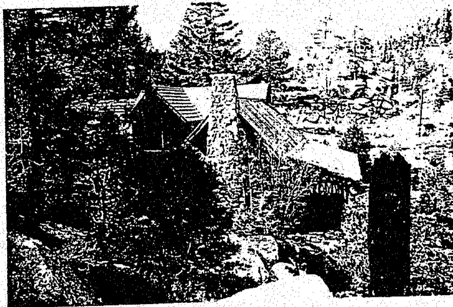
Cabin No. 68, view looking west showing newer addition at left
