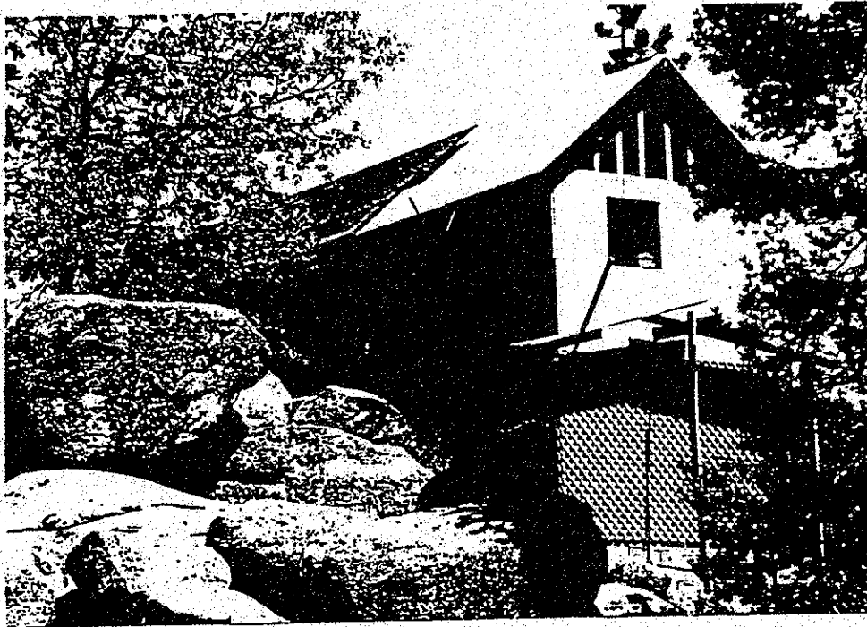
Cabin No. 63, showing addition under construction (August 1989)
