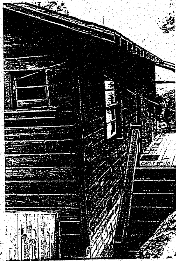
Cabin No. 55, view looking east
