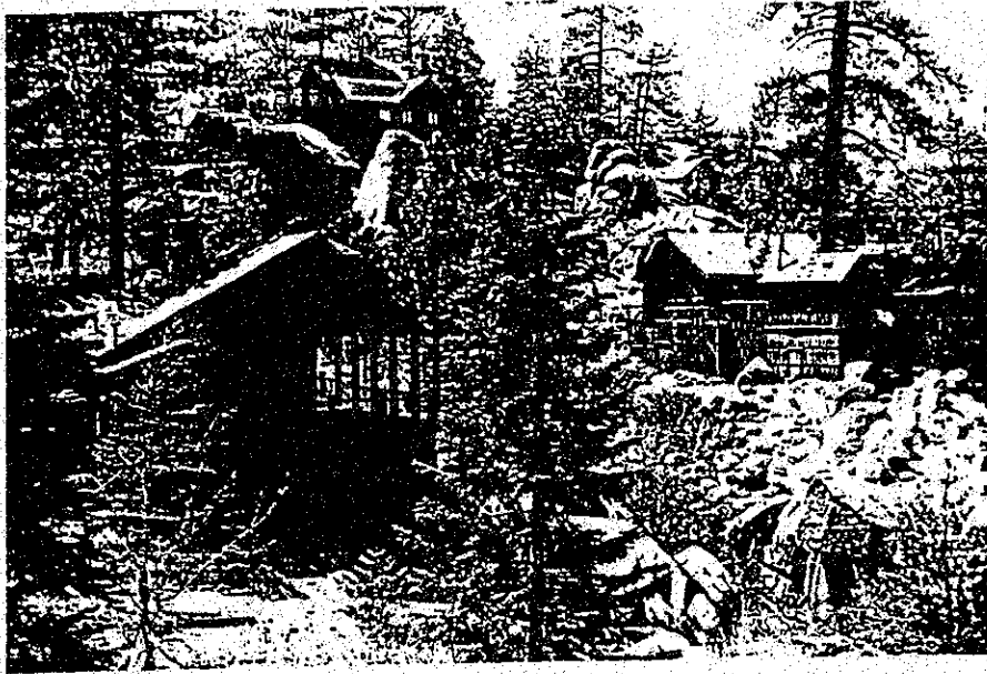
View looking southwest at Cabins 85, 77 and 57, Kidd Cove
