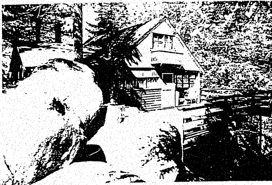
Cabin No. 43, showing original cabin at left
