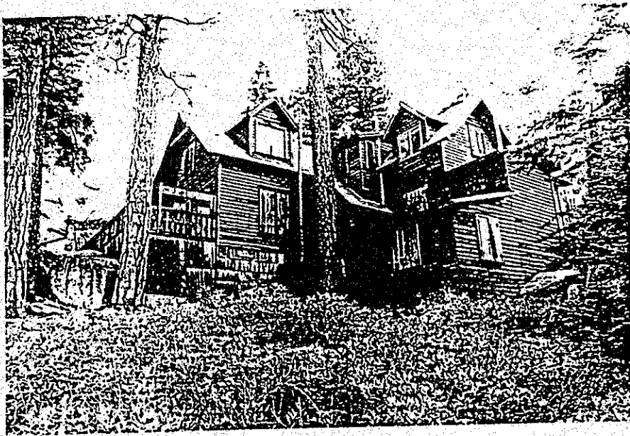
Cabin No. 62, view looking southeast
