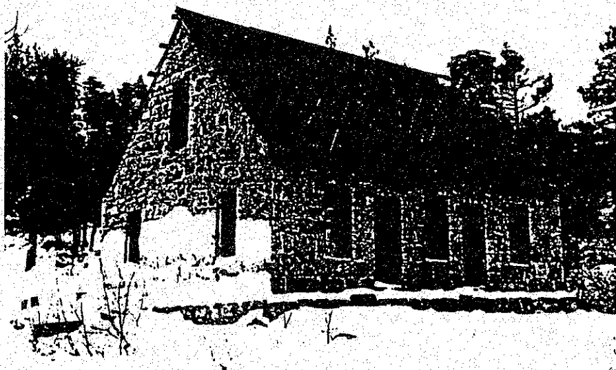
Dam Keeper's House (1987), View Looking West
