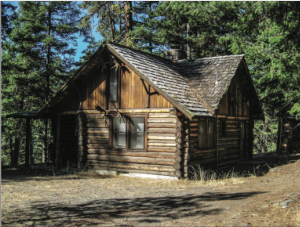
Figure 22—This 1948 recreation residence in the Hart Creek tract at the Okanogan-Wenatchee National Forest in the Pacific Northwest Region was built close to the ground on a concrete foundation. The low foundation has not led to deterioration of cabin logs because the climate is relatively dry and the soil drains well.
