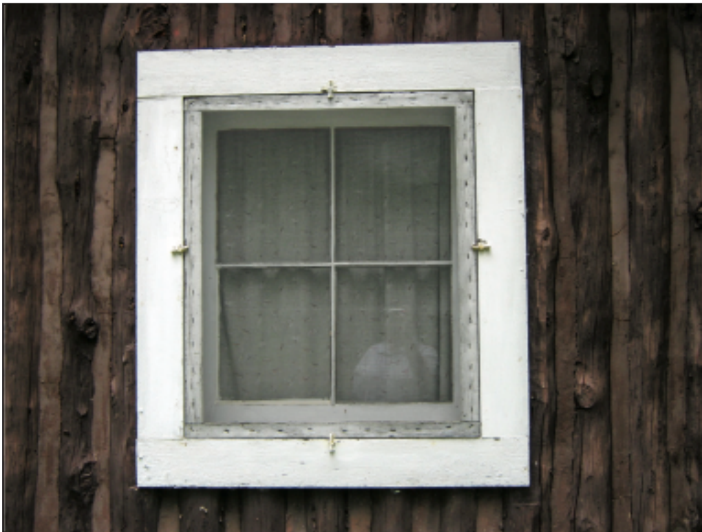
Figure 15—The screen on this small divided-lite window keeps bugs out when the window is open during the summer. The screen is attached using four pivoting double wing screen clips for easy removal. The 1958 recreation residence is at the Rollways tract of the Huron-Manistee National Forest in the Eastern Region.
