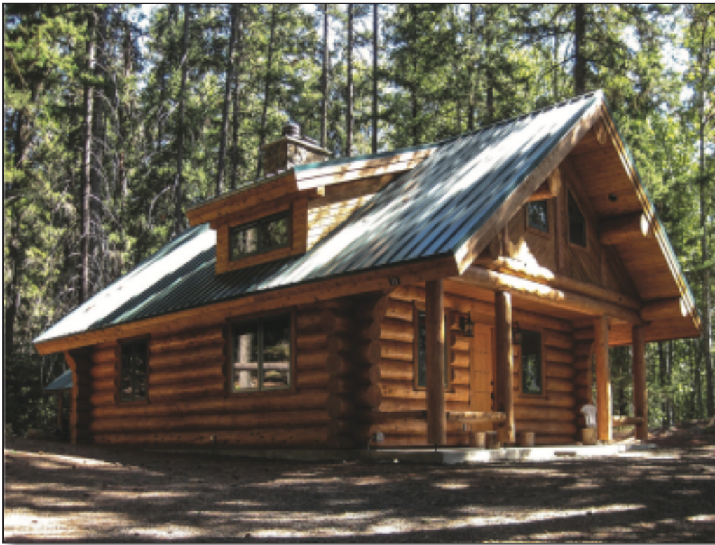
Figure 35—This replacement recreation residence at the Okanogan-Wenatchee National Forest’s Indian Creek tract in the Pacific Northwest Region was built in 2006. The size, general shape, proportions, window-to-wall ratio, colors, and materials are reasonably similar to historic residences in the tract, but the design doesn’t mimic the historic buildings.
