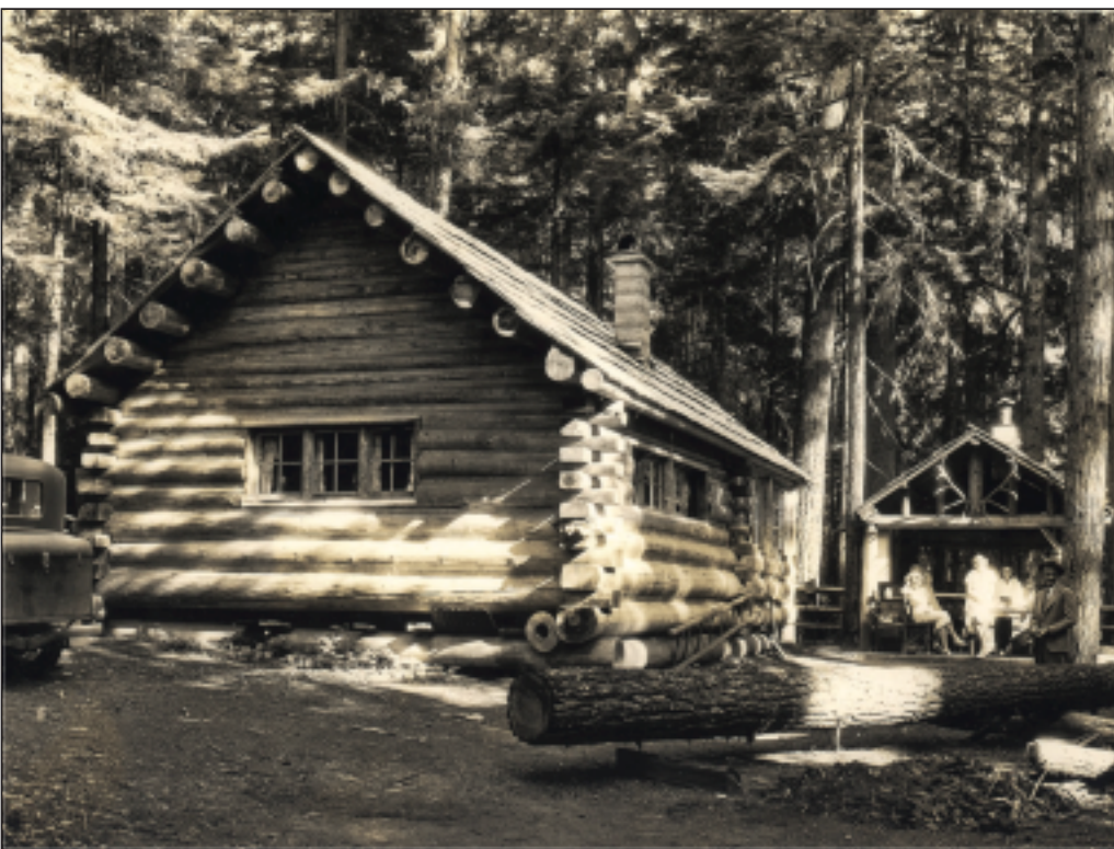
Figure 27—This early 20th century photo shows a family enjoying a covered outdoor room next to its recreation residence at the Silver Springs tract of the Mt. Baker-Snoqualmie National Forest in the Pacific Northwest Region. The outbuilding was built about the same time as the residence with similar materials in a similar style.
