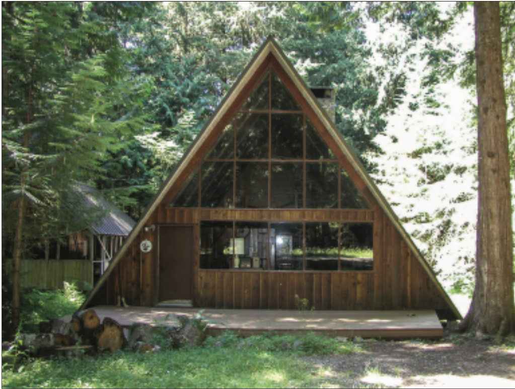
Figure 1—This 1961 A-frame recreation residence contributes to the historic Dalles tract of the Mt. Baker-Snoqualmie National Forest in the Pacific Northwest Region. Although this is a newer style than usually comes to mind when considering historic recreation residences, it was popular in the region during the 1950s and 1960s. There are five A-frames in this tract; this one still looks the same as when it was built.
