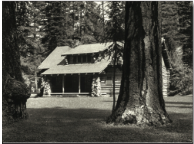
Figure 28—This 1938 recreation residence is surrounded only by native vegetation at the Moore's Creek area of the Boise National Forest in the Intermountain Region.
