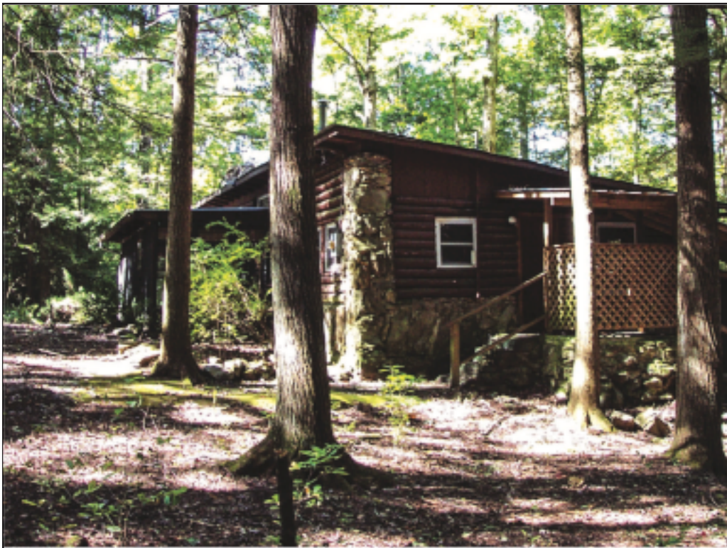
Figure 14—Natural stone was used at the corners, on the lower portion of the walls, and as the foundation for this recreation residence at the Pisgah National Forest in the Southern Region.
