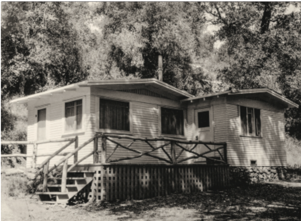
Figure 2—This recreation residence in a riparian canyon of the Cleveland National Forest in the Pacific Southwest Region has character-defining features typical of that area in the 1920s: a distinctive low-slope roof with exposed rafter tails, rock foundation, narrow beveled lap siding, rustic pole railings, perpendicular lattice under the porch, and removable screens on each window.
