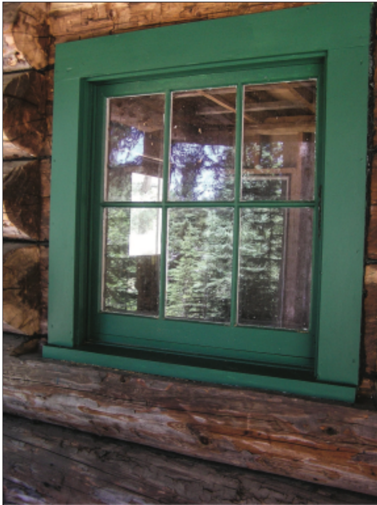
Figure 6—This window on a cabin at Adams Camp of the Nez Perce National Forest in the Northern Region was rebuilt to match the historic window, installed in the original window opening, and painted the original color. Window replacements that match the historic windows are minor changes.
