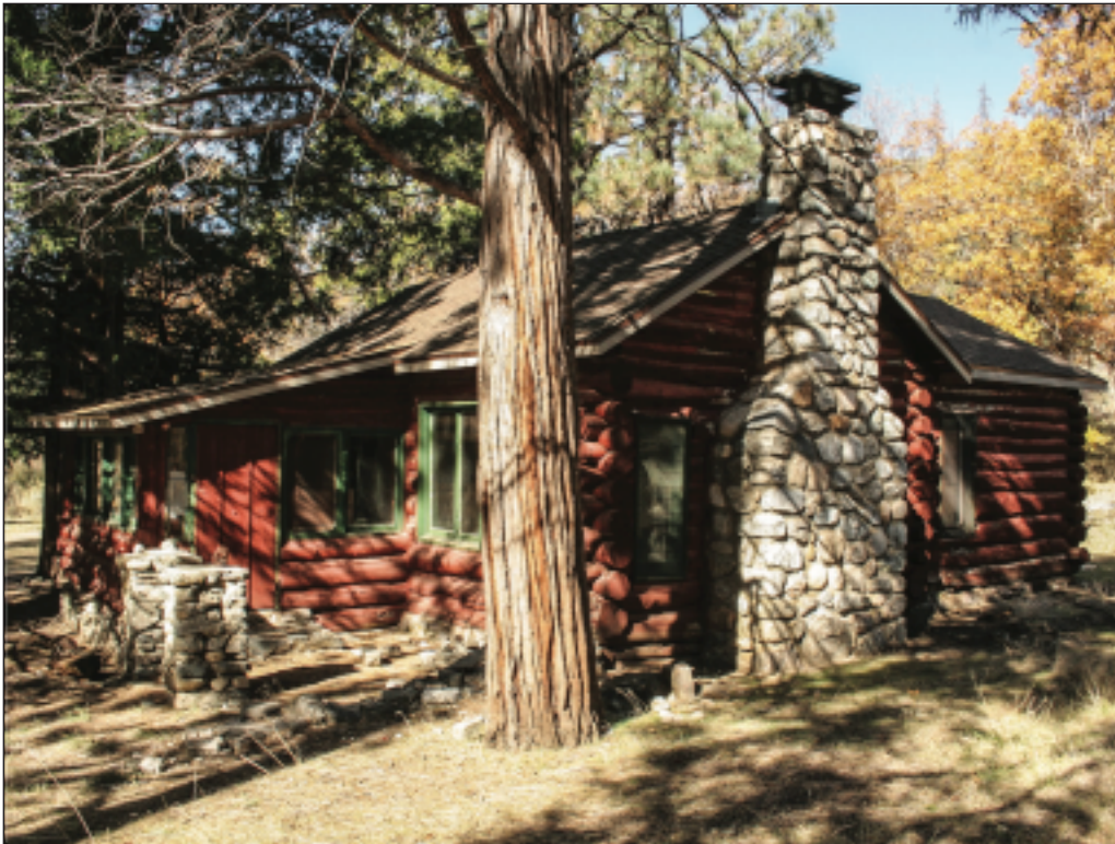
Figure 30—Located at the Seven Oaks tract of the San Bernardino National Forest in the Pacific Southwest Region, the addition on the back of this log recreation residence is compatible in size and construction.
