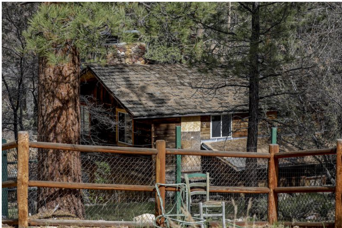
Wooden roof shingles and pine trees near homes increase the fire danger in the community of Sugarloaf, near Big Bear Lake. (Irfan Khan / Los Angeles Times)
